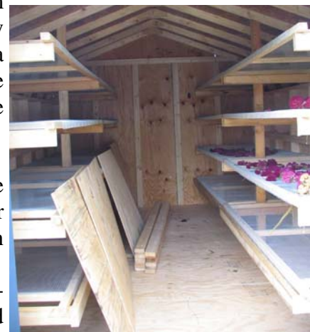
Inside of an herb dryer, constructed for the Medicinal Herbs for Commerce Project
